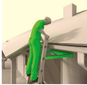
Figure showing use of a stand-off device to ensure a strong resting point.
