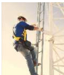
Ladder equipped with anchorage railing.
