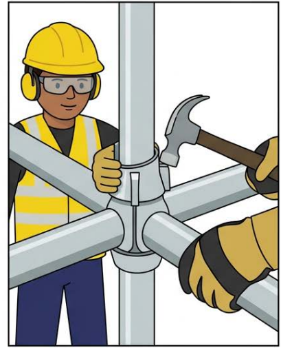
3- Tighten with hammer blow.
